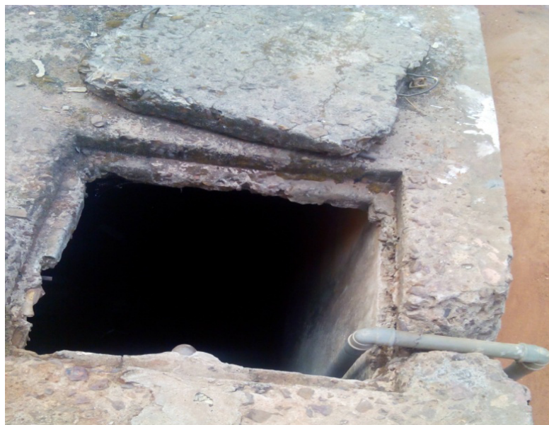
Figure 5: BOREHOLE HEAD AT PERM. SITE
