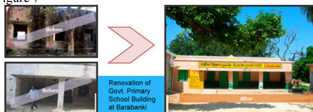
Fig. 7: Rehabilitation assistance (Source: POWERGRID of India)
