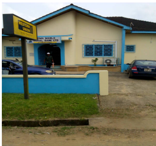
Photo credit: Author Front view of main office
