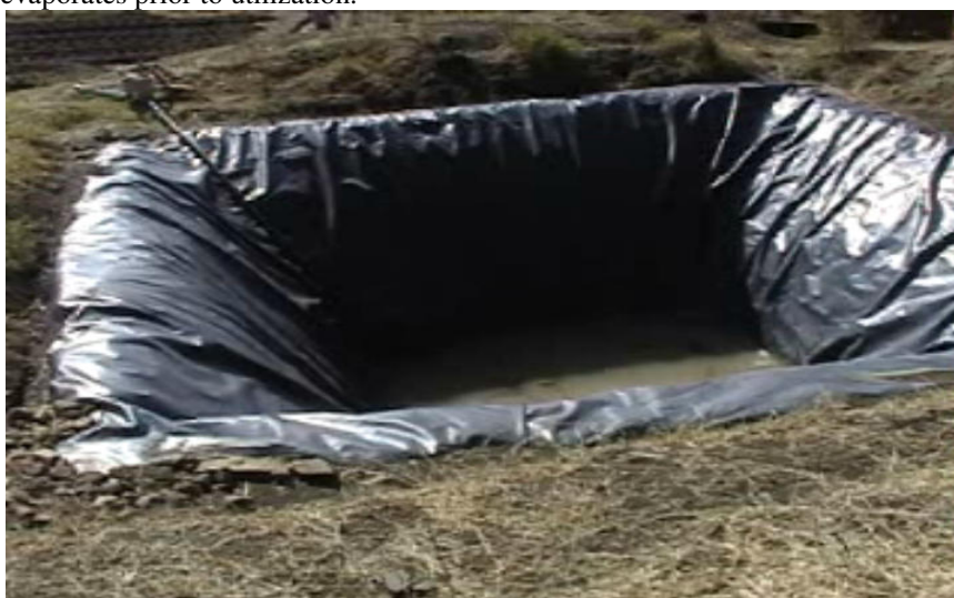
Plate 1 Trapezoid geomembrane for harvesting rain water.
