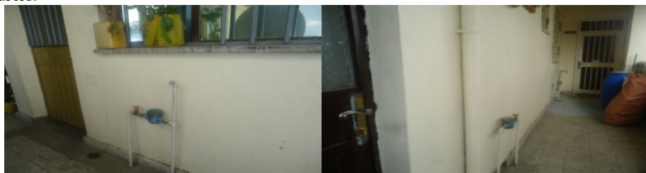
Figure 3: Residents' Own Private Tap at the New Settlements, Gotera and Gofa Mebrathaile Condominium Houses
