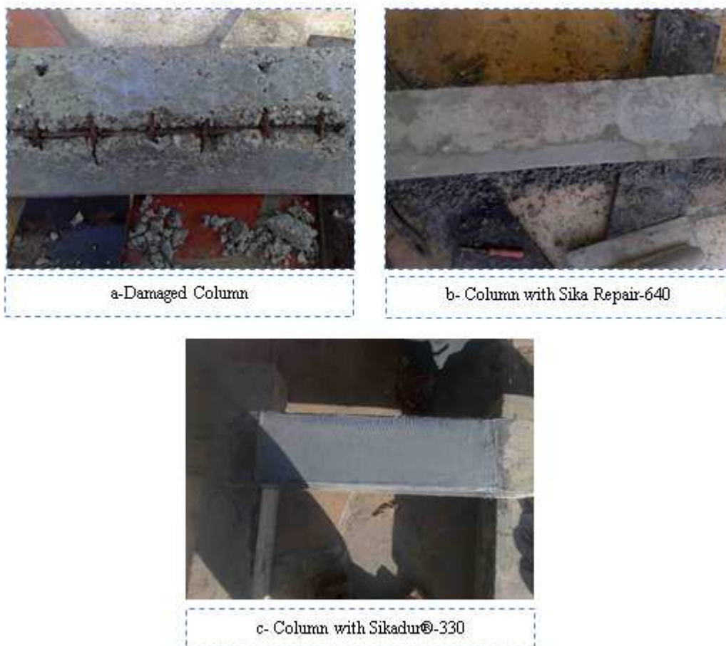
Fig 9. Repaired of Columns
