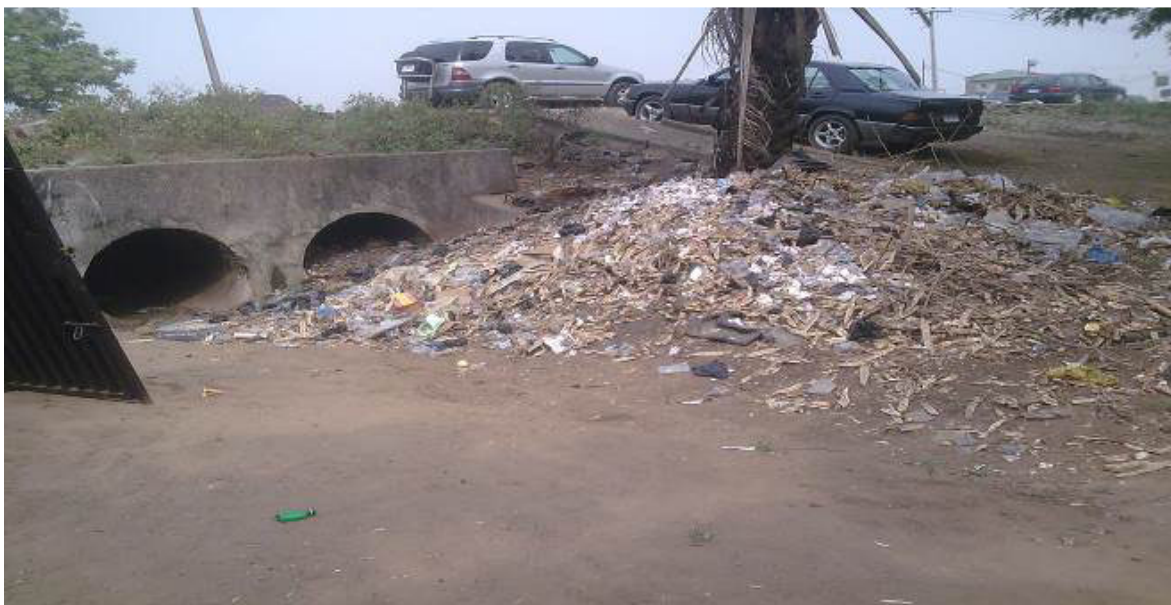
Figure 5. Drainage canal converted to welder's workshop.
