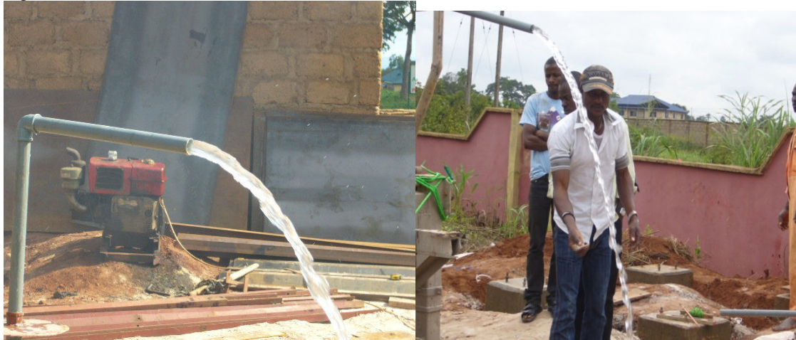
Figure 2 a and b pump testing of borehole water
