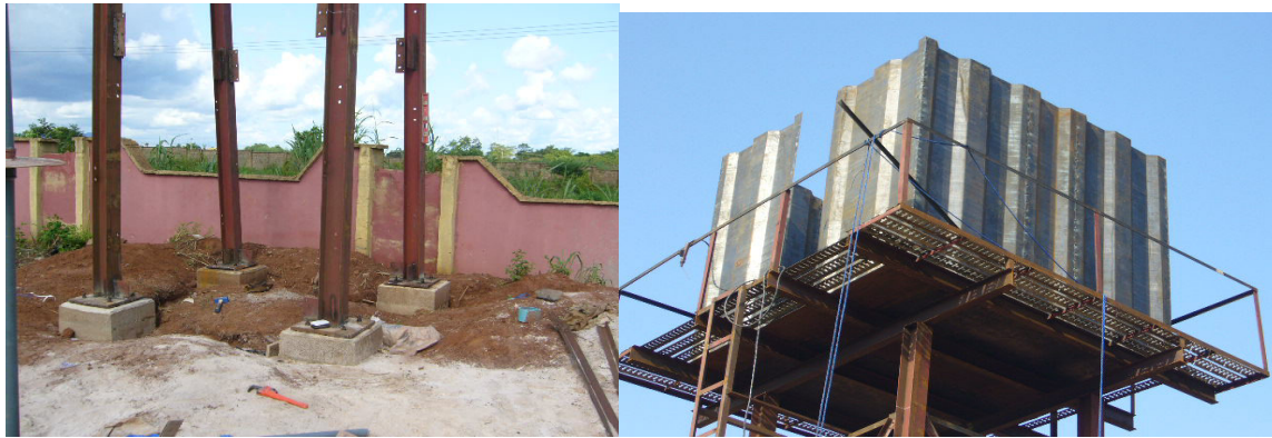
Figure 2 a and b stanchion stands and overhead tank under construction
